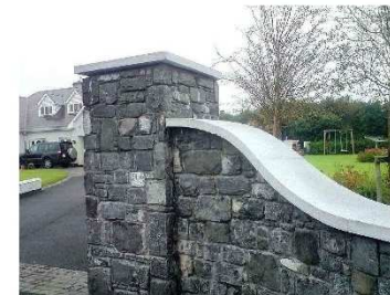
GRANITE STONE WALLS.
